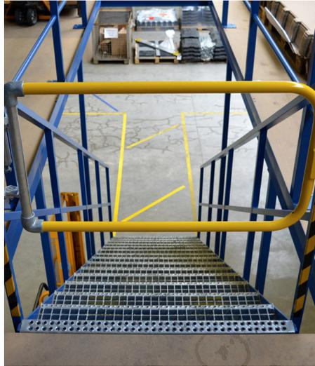
and overcoming the potential for human error. This type of system is the preferred solution to chains, bars or sliding tubes, as these traditional forms of protection can lead to a hazardous void, when used incorrectly.
